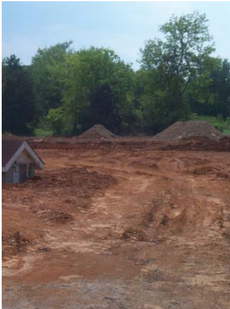
Site preparation begins for the Primary Care & Hope Clinic.
